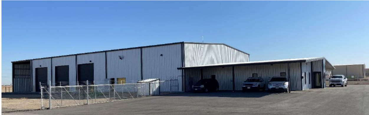
Midland, Texas pin-to-pin manufacturing facility.
